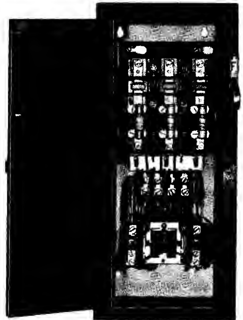
G-E CR7008 combination a-c magnetic starter with cover open
